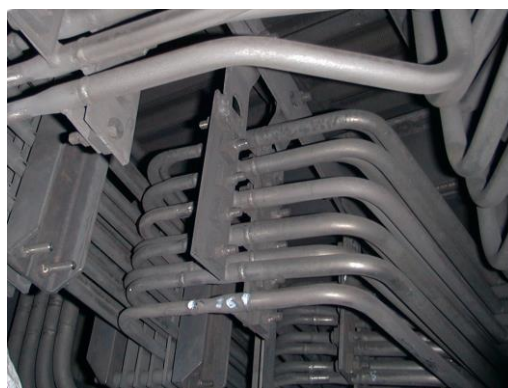
View of a bank of economiser tubes situated ~6 metres above the floor of the SBA
